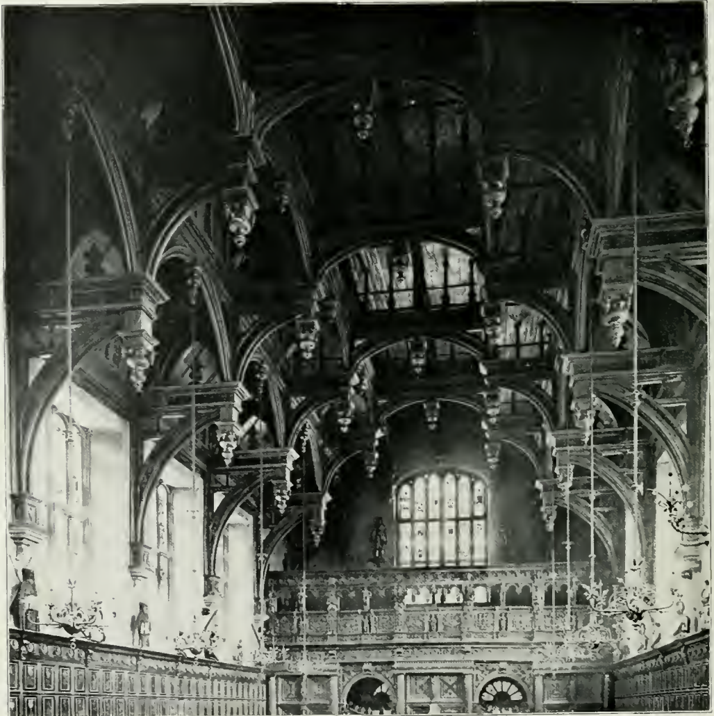
OPEN TIMBER ROOF, MIDDLE TEMPLE HALL, LONDON
